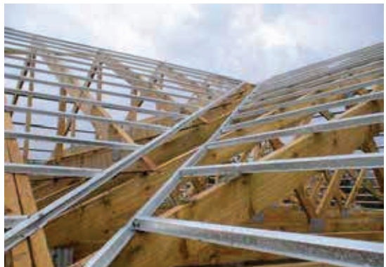
STEEL PURLINS ON TIMBER ROOF
