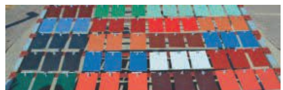
MRM corrosion site at Mariakani, Mombasa
