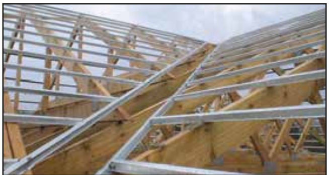
STEEL PURLINS ON TIMBER ROOF
