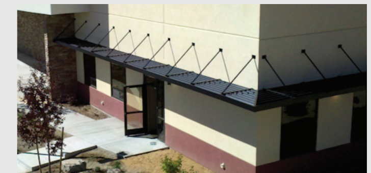
Sun shading devices including full-façade shading.
